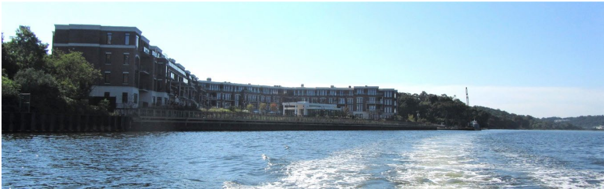
The Residences at Glen Harbor development close to completion on eastern shore of the harbor in Glenwood Landing (photo by Carol DiPaolo, 8/24/22)
