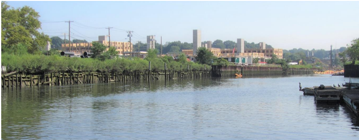
Garvies Point development project along north side of Glen Cove Creek, view looking east toward head of the creek (photo by Carol DiPaolo, 8/29/18)
