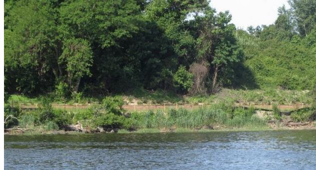
Wetland-restoration planting at Bar Beach lagoon in 2003 (above, l) and in 2005 (above, r) (photos by Kevin Braun) and view of west shore and construction of the Town of North Hempstead trail (r) (photo by Carol DiPaolo, 6/17/20)
