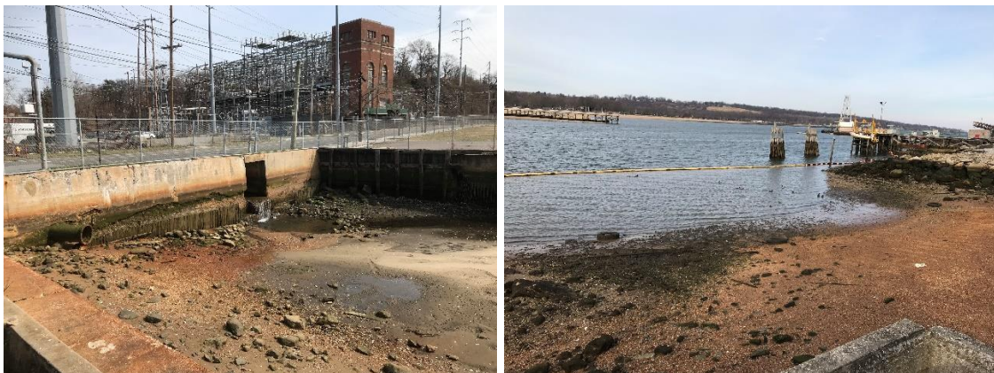
Powerhouse drain (CSHH #14A) at low tide (l) and view looking north west beyond adjacent fuel terminal dock (r) (photos by Michelle Lapinel McAllister, 3/20/20 and 5/27/20, respectively)
